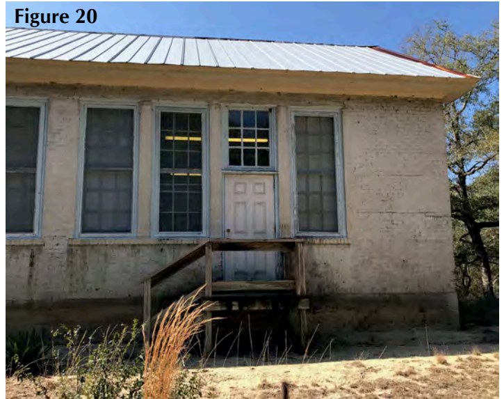
Modern door added to the east elevation of the building
