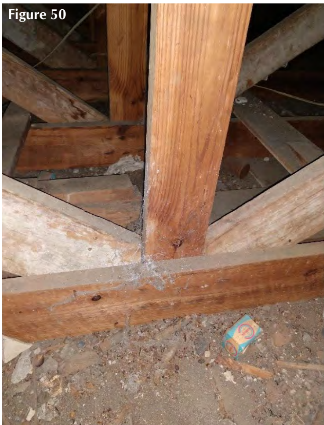
Typical roof truss brace connection
