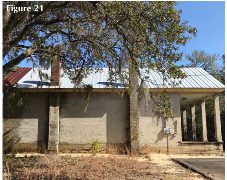
The west elevation of the building
