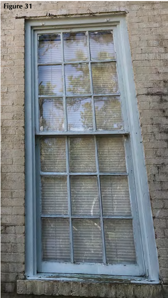
Typical window, exterior view
