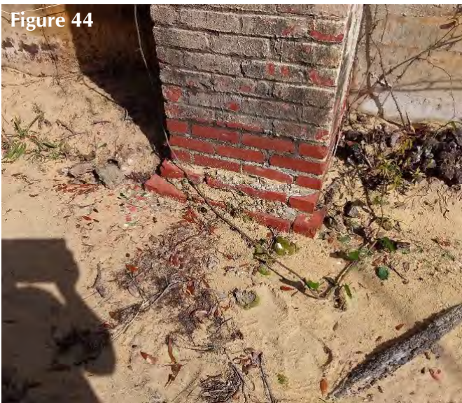
Chimney sitting on exposed masonry foundation
