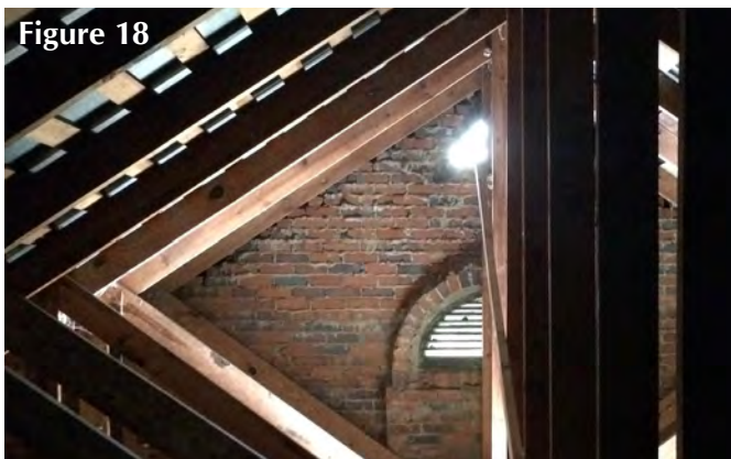
Attic masonry showing 1 wythe thick pediment
