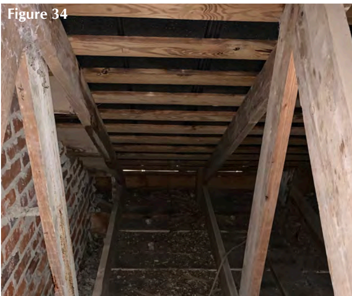
Notice plank roof sheathing and no insulation
