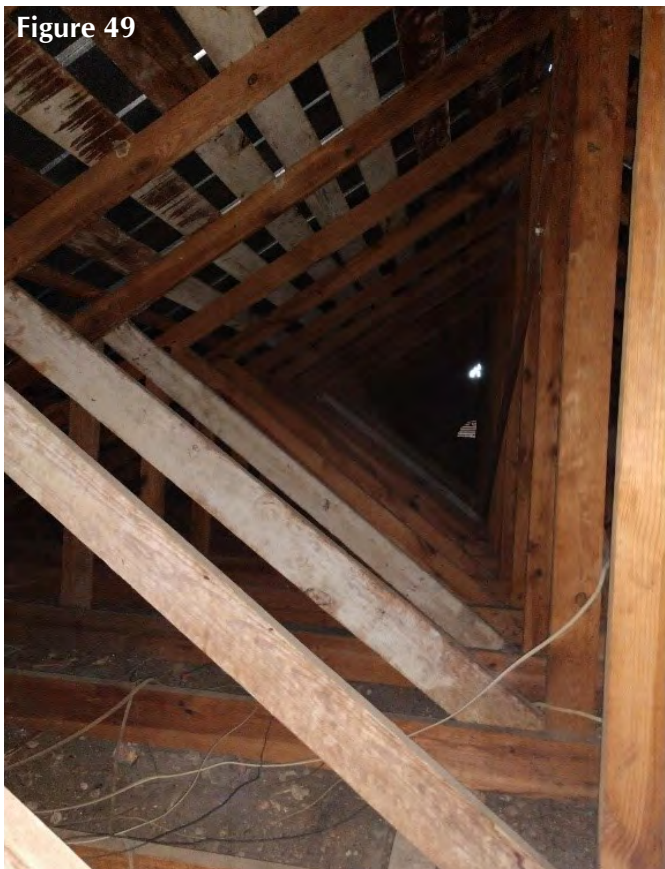
Typical roof framing rafter and brace
