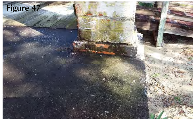
Figure 47 Masonry column sitting on porch slab
