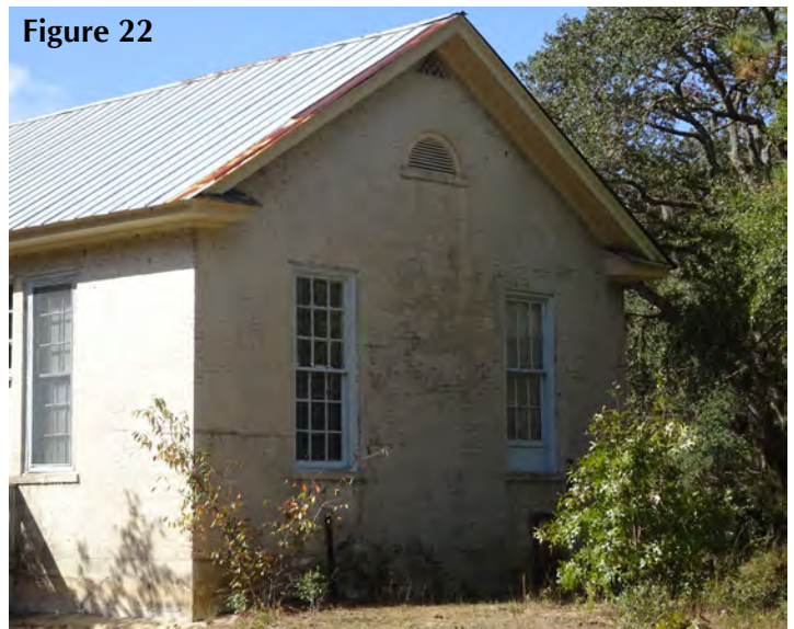
The north elevation of the building
